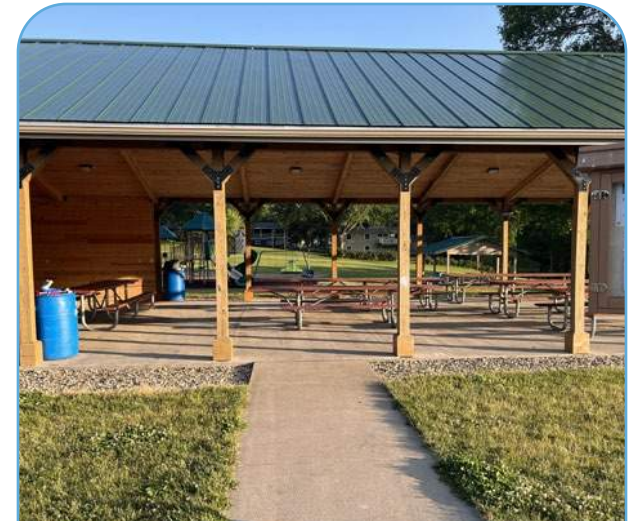
Main Shelter at Putnam Park
