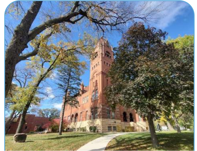
Faribault County Courthouse
