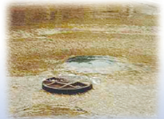
Collection system overflow due to infiltration and inflow
