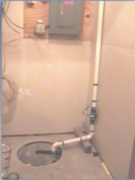
Properly Installed Sump Pump
